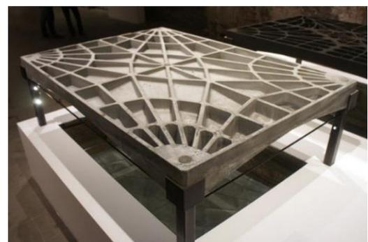
Figure 4: Material efficient floor slab (Block research group, ETH Zurich)
